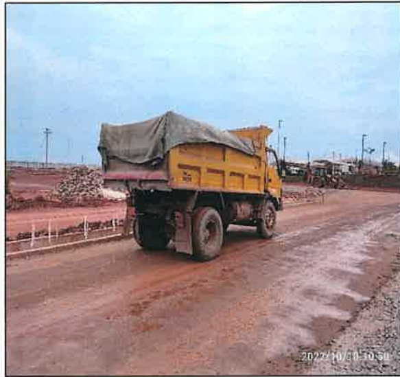
CONSTRUCTION / EXCAVATED MATERIALS TRANSPORTED BY COVERING WITH TARPULIN SHEETS
