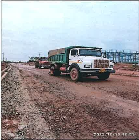
CONSTRUCTION / EXCAVATED MATERIALS TRANSPORTED BY COVERING WITH TARPULIN SHEETS
