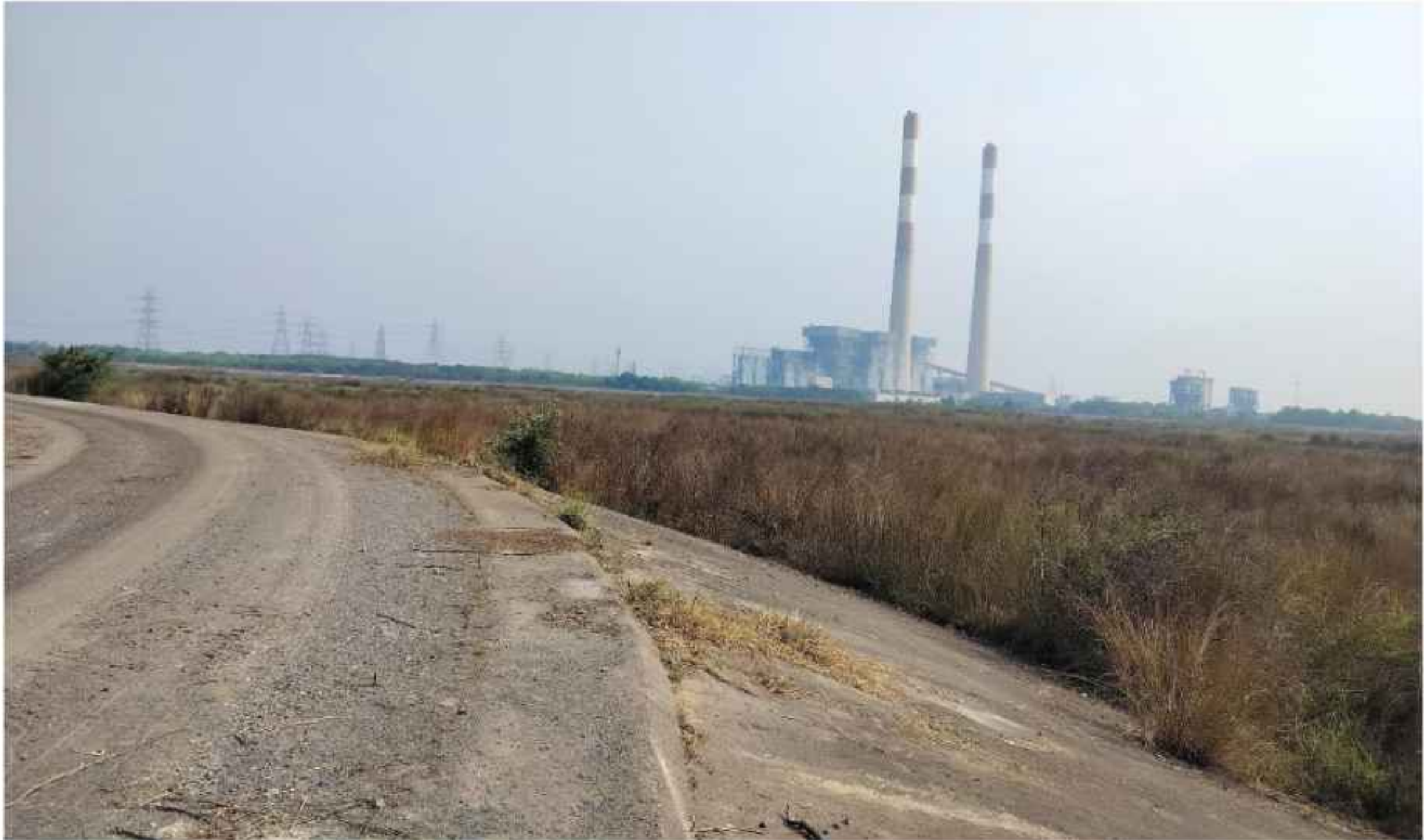
PHOTOGRAPH-3, ROAD OVER DYKE & UPSTREAM SLOPE LINING
