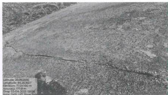
Exposure of Geomembrane at Intersections on U/S Slope
